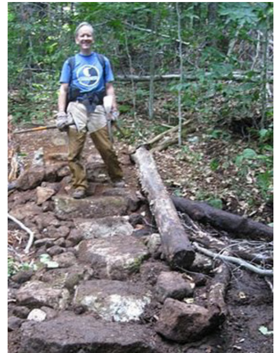
Trailwrights members attending to erosion control, rock steps and trail hardening on the Pemigewasset trail at Franconia Notch State Park last summer.
