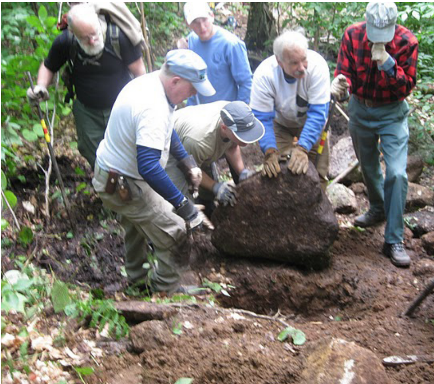
Trailwrights members attending to erosion control, rock steps and trail hardening on the Pemigewasset trail at Franconia Notch State Park last summer.
